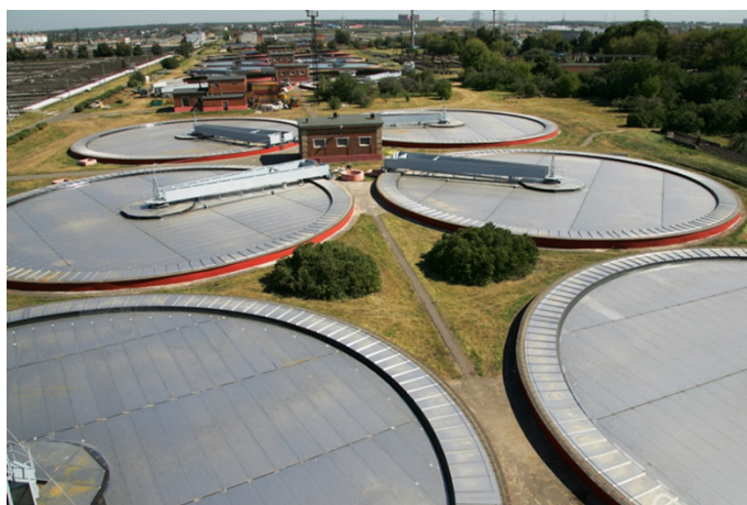
Lyubertsy wastewater treatment in Moscow, Russian Federation (Mosvodokanal, 2020)
