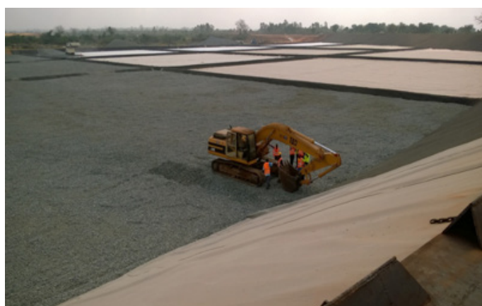
Aképé Sanitary landfill, 1st disposal at the new treatment site Inauguration 28 Jan 2018
